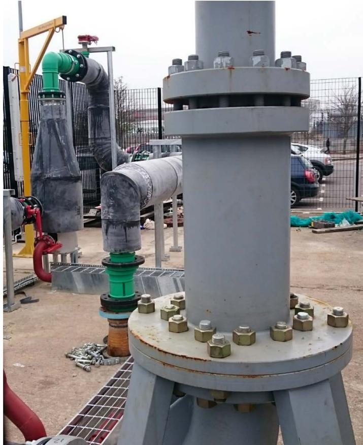
Figure 1. Well head at the Southampton geothermal site.
