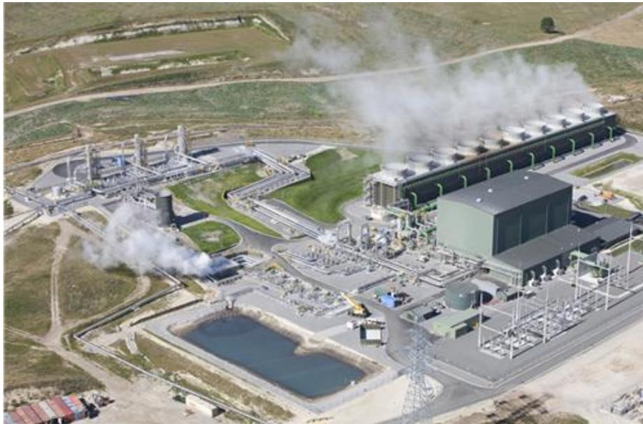
**Figure 1.** Nga Awa Purua (Rotokawa) 140 MWe power plant, the world's largest triple flash single geothermal turbine (commissioned April 2010).
