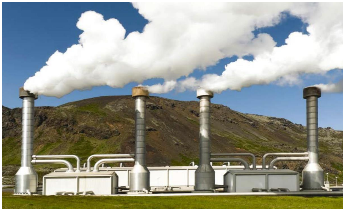
Figure 12.1 Nesjavellir geothermal power plant.
